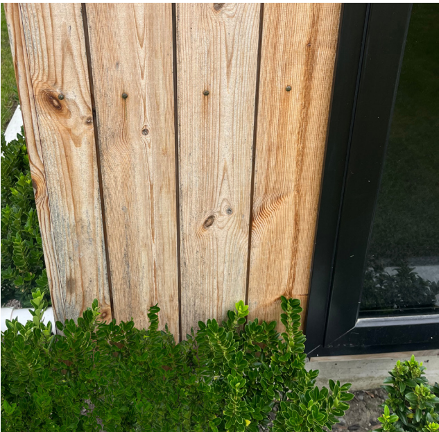
Vegetation too close to the weatherboards, restricting airflow, retaining moisture, and obstructing access for future maintenance.
