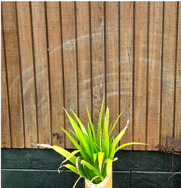
Signs of wear from vegetation contact—this cladding surface was scratched by nearby plants.
